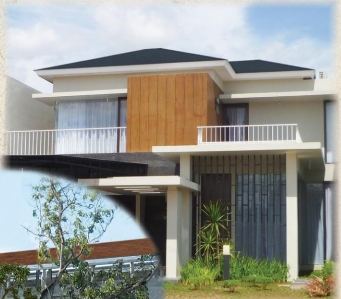
BITURUV REGULAR PATTERN CB : Diamond Black CITRA GRAND CITY PALEMBANG Sumatera Selatan
