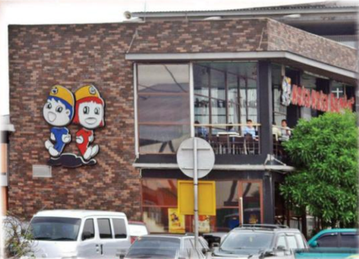
TERRA CEDAR (w/ Grouting) HOKA - HOKA BENTO, Rest Area Km. 19, Bekasi.
