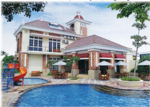
TERRA GOLDEN (w/o Grouting) ROYAL RESIDENCE, Pulo Gebang, Jakarta Timur.
